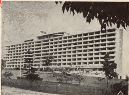
In contrast to the rugged, forbidding architecture of most northern hotels, the El Panama is built for maximum air and sunshine.
